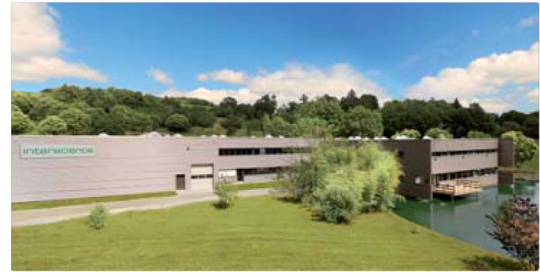
interscience R&D center and manufacturing plant Mourjou FRANCE
